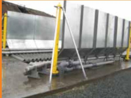
InterClean designs the wash system to handle the effluent and manage extreme amounts of mud removed from the vehicles. Large settling pits and filtration assures we are providing high quality wash water.
